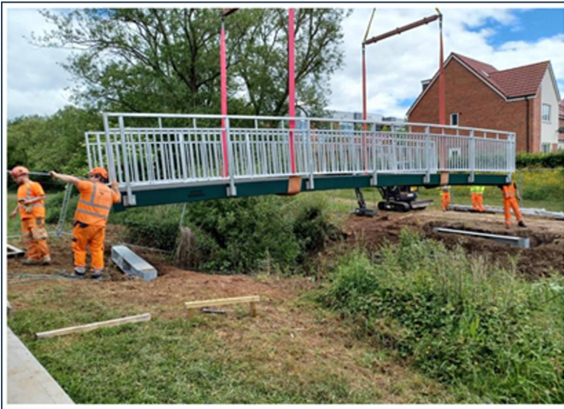
Figure 1-2 - Example Bridge Construction
